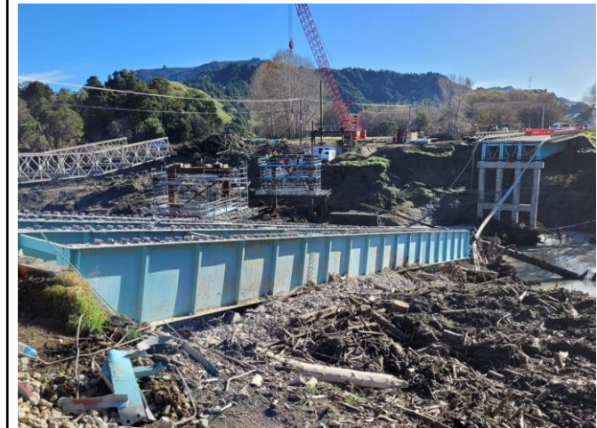
6 June 2023: Hikuwai Bailey bridge under construction
