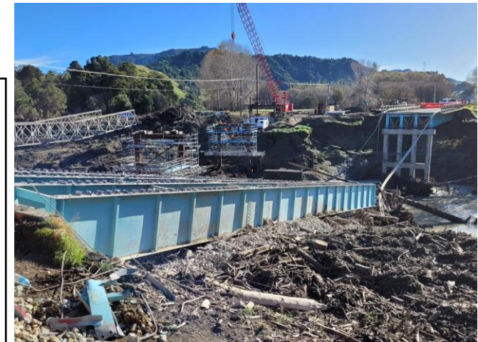
6 June 2023: Hikuwai Bailey bridge under construction
