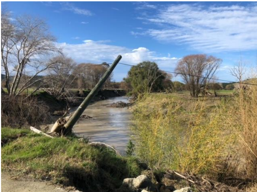
A power pole knocked over on Paroa Station in Tairāwhiti.
