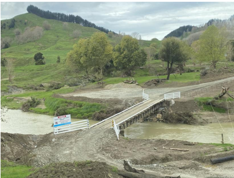
The image shows the bailey bridge at Bushy Knoll through the Blue Berry Flats (in Tairāwhiti). The load limit is 3500kg and it is well used by the local rural community.
