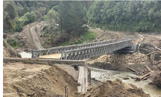
5 May 2023 A Bailey bridge now spans Waikare Gorge
