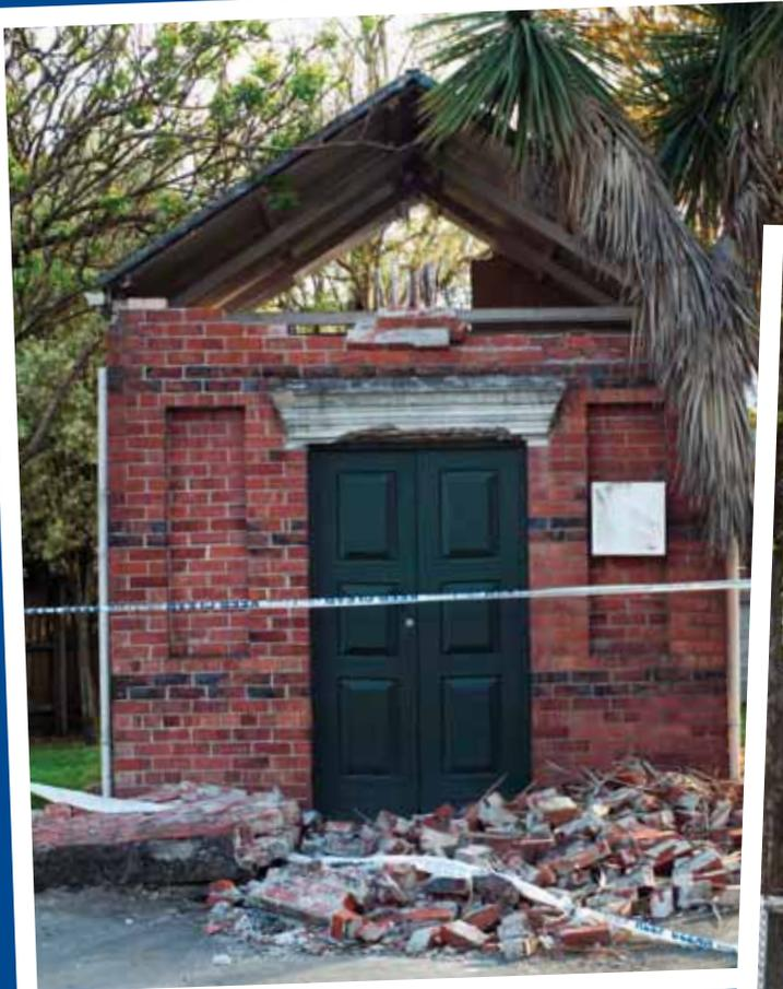
^ This electricity substation had been decommissioned prior to the earthquakes and was unstrengthened
