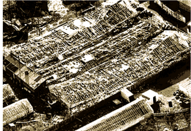
WIND DAMAGE Photo: Christchurch Press . Damaged glasshouses after a severe windstorm, Christchurch, July 1995.
