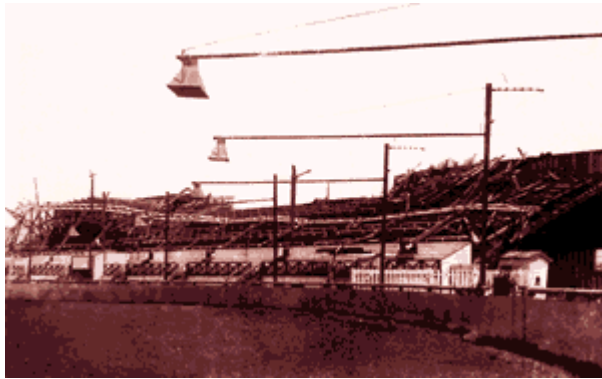
STORM DAMAGE Photo: New Zealand Free Lance Collection, Alexander Turnbull Library, Wellington, NZ. Remains of the members' stand at the Show Ground, Palmerston North, February 1936.
