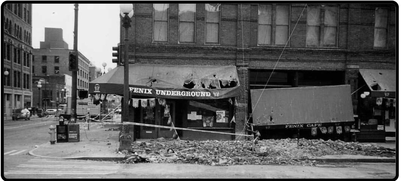
The brick parapet over the Fenix Cafe in Pioneer Square, Seattle, collapsed in rubble during the earthquake on 28 February.
