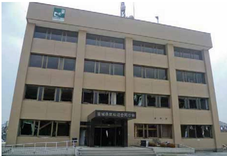
Example of a successful designated tsunami evacuation building in Kesenuma, Miyagi Prefecture, Japan. This office building was inundated to a height of 8 metres and sustained minor scour and non-structural damage. Videos show that people survived on the roof of this building.
