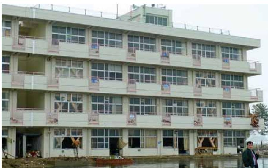
Arahama Elementary School, Miyagi Prefecture, Japan. Located 750 metres from the coast, this building was successfully used as a refuge for 380 schoolchildren and surrounding residents in 7.5-metre deep inundation. The building suffered non-structural damage from water flow and debris impact.
