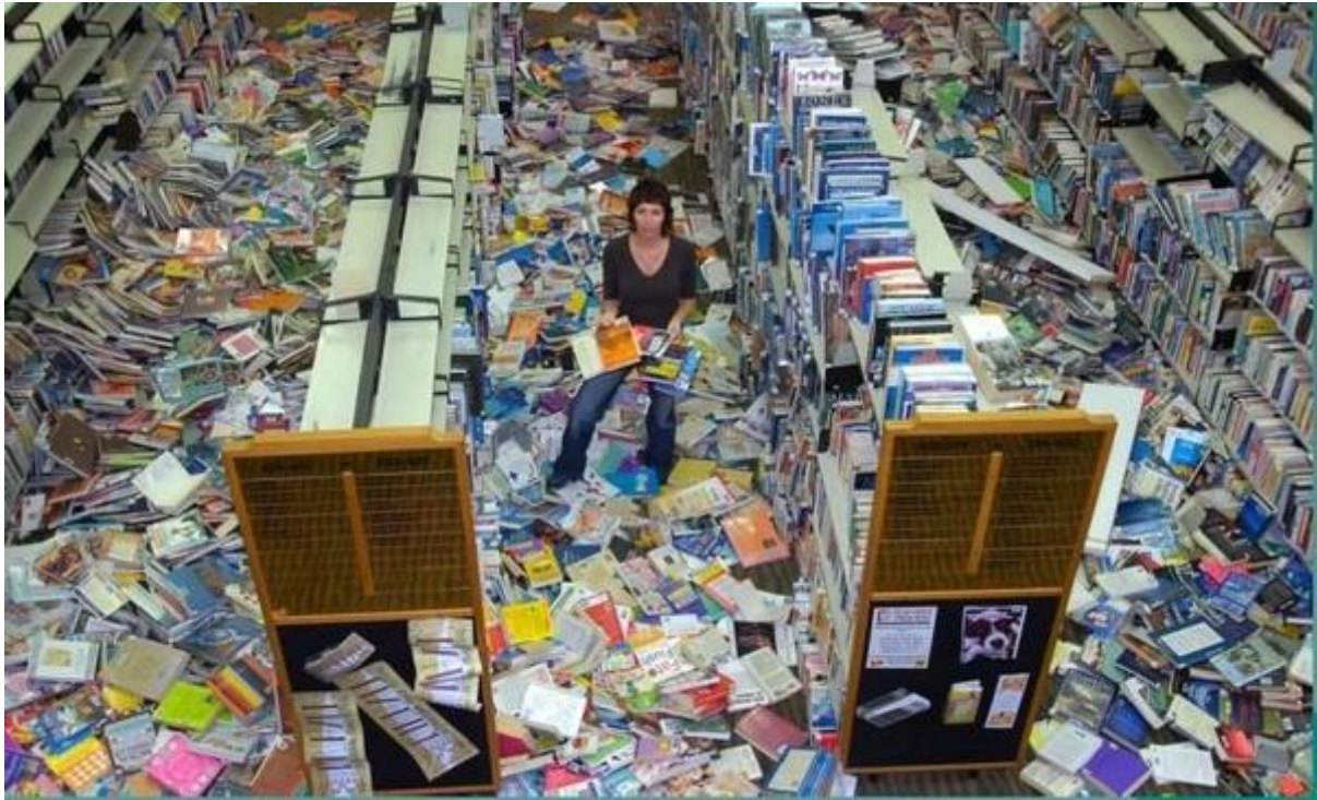
Earthquake damage to HB Williams Memorial Library. Photo courtesy Gisborne District Council.
