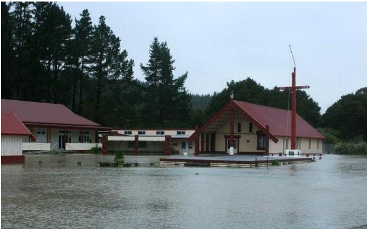
Flooding at Otiria Marae, Northland. Photo courtesy Far North District Council.
