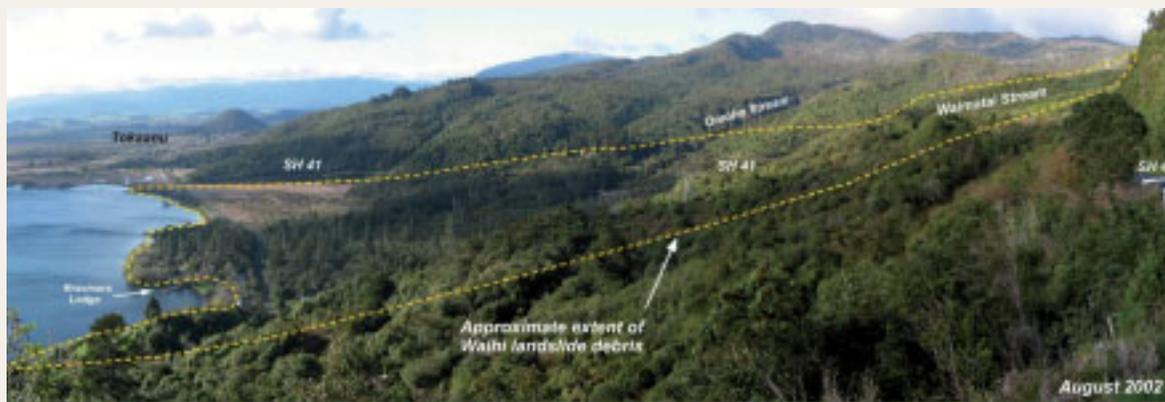
Several large landslides, which have formed very large debris flows, have occurred at the Hipaua Steaming Cliffs on the Waihi Fault scarp at the southern end of Lake Taupo over the last 230 years.
