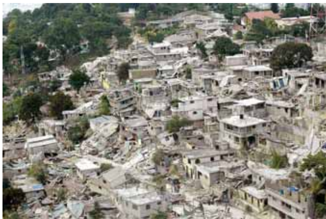
Left: The 2010 Haiti earthquake resulted in the collapse of around 70 per cent of regions buildings killing more than 200,000 people.
