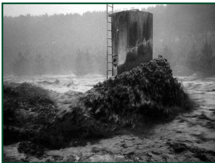
Back in 1995, the Trans Rail lahar tower takes a pounding as the lahar roars down the Whangaehu river.
