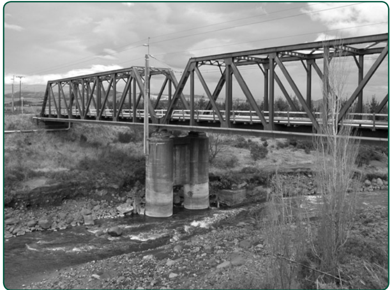
In the extreme event scenarios, travel times for the lahar to the Tangiwai bridge are around 90 minutes with expected peak flows of up to 1800 cubic metres per second. This would place the bridge at risk.
