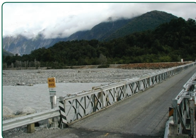
Flood defences on the true left bank that provide protection to the holiday park area – the raised glacier access road and rock groynes upstream of SH6
