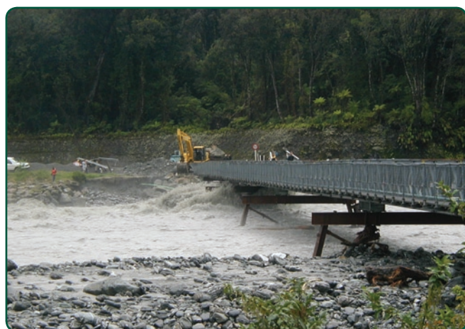
Maintenance work on the SH6 bridge
