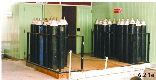
Inadequately restrained gas cylinders at A & E (see Table 6.1)
