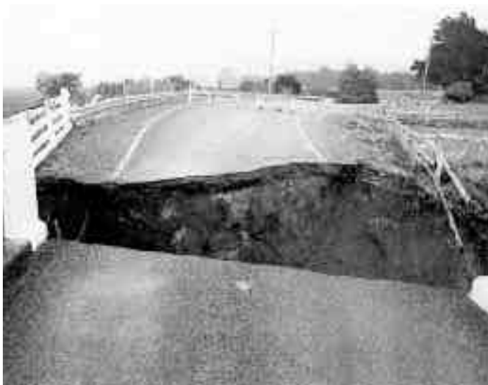
Figure 4.13. Mangatarere Bridge, Belvedere Road, Carterton District. The road was closed in November 1994 when the western bridge approach was eroded. Photo courtesy of the Wairarapa Times-Age.
