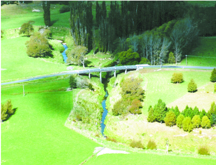
Figure 4.5. The Tinui Bridge on the Masterton-Castlepoint Road. This single lane structure is sited on an area of high liquefaction potential.
