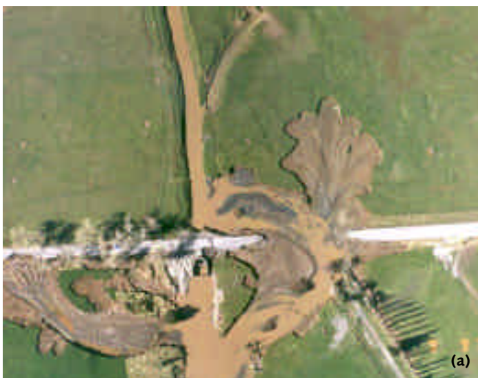
Figure 4.13. Mangatarere Bridge, Belvedere Road, Carterton District. The road was closed in November 1994 when the western bridge approach was eroded. Photo courtesy of the Wairarapa Times-Age.
