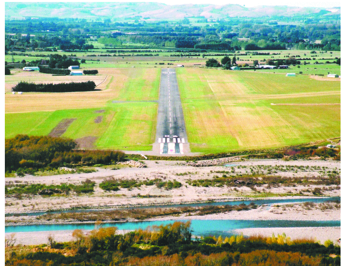
Figure 4.16. Southern end of the Hood Aerodrome runway, Masterton. Severe erosion occurred in 2000, reducing the 'over-run' area and threatening the runway. Extensive river realignment and rip rap protection was required.
