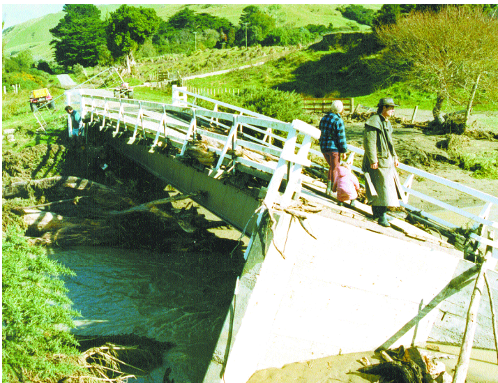
Figure 4.12. Damage to the Packsur Bridge, Mataikona, following scouring and rotating of the abutments in April, 1991.
