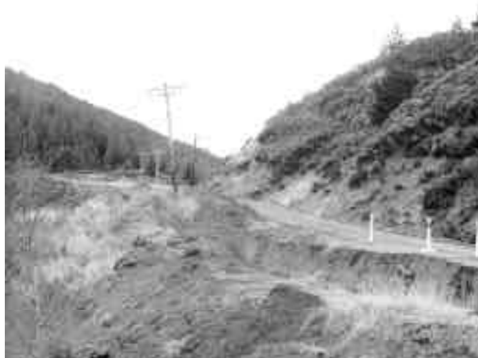
Figure 4.7. Masterton Castlepoint Road at the Whakataki Saddle. This important route was severely affected by slumping in August 1974.
