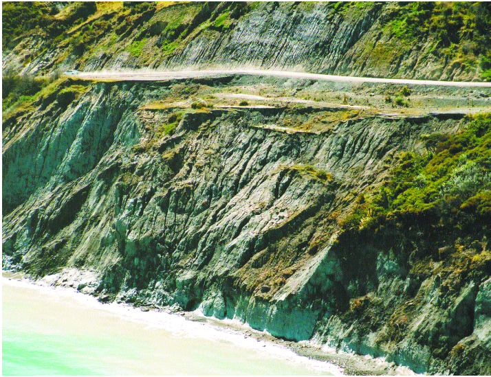
Figure 4.10. Cape Palliser Road at Te Kopi. There is severe instability of the road at this location due to coastal erosion and slumping of the mudstone material. Note the succession of previous road levels below the present road.
