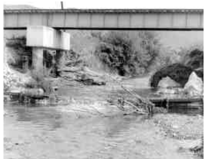
Figure 4.15. The rail bridge at Abbots Creek, Featherston. In November 1975, rockwork and a weir were installed to counter bed-scour at the piers.
