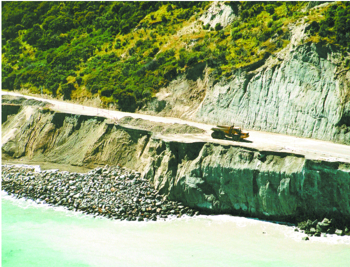
Figure 4.11. Cape Palliser Road at Whatarangi Cliffs. A boulder beach is under construction to counter severe beach erosion.
