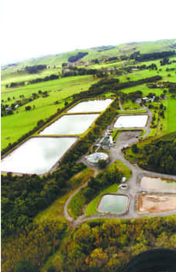
Figure 3.4. The Masterton water treatment plant at Upper Plain. The three water ponds are on the left of the picture and the clear water pond is in the foreground. The clarifier is in the middle of the picture and the filters and treatment plant building are above the clarifier.
