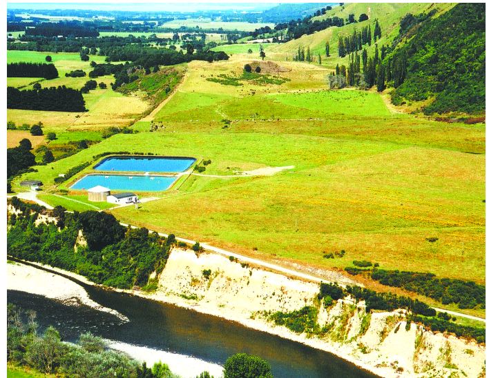
Figure 3.6 Waiohine River intake to Moroa water race and Greytown/Featherston water supply. The filtration plant and storage ponds are sited to the west of the Wairarapa Fault.
