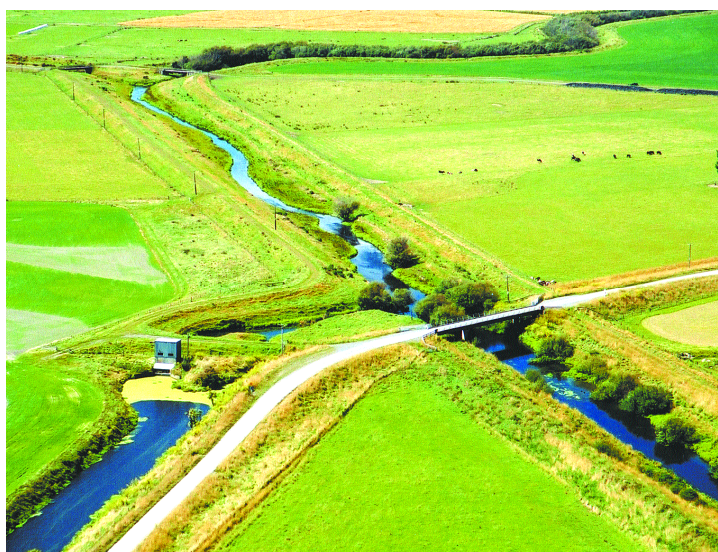
Figure 3.20. Pouawha pump station in the Lower Wairarapa Valley. Twin electric pumps lift the water from the low-lying former Pouawha lagoon.
