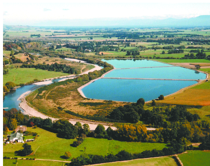
Figure 3.10. Masterton sewage treatment ponds at Homebush. The two primary ponds are in the foreground and the secondary pond and discharge are in the background.
