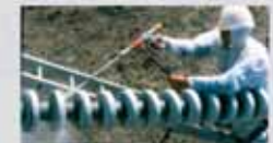
Ash is removed from a 110 kV insulator tower using pressurized water following the 2003 Taupo eruption, New Zealand (Teapouran, New Zealand).
