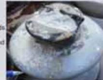
Insulator covered in 132kV insulator following the May 2008 Clarendon eruption, UK.
