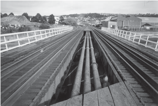
Oil Pipelines from Oil Wharf to Storage Tanks Crossing Leith Rail Bridge - BP Oil Limited
