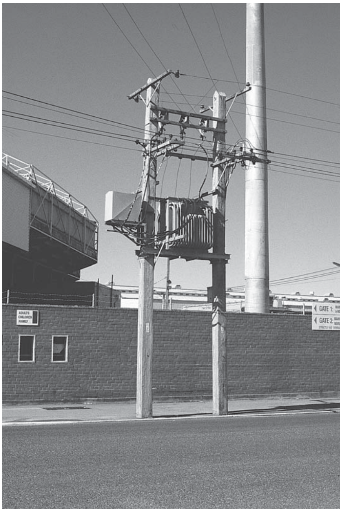
Typical Pole Mounted Transformer - Civil Defence
