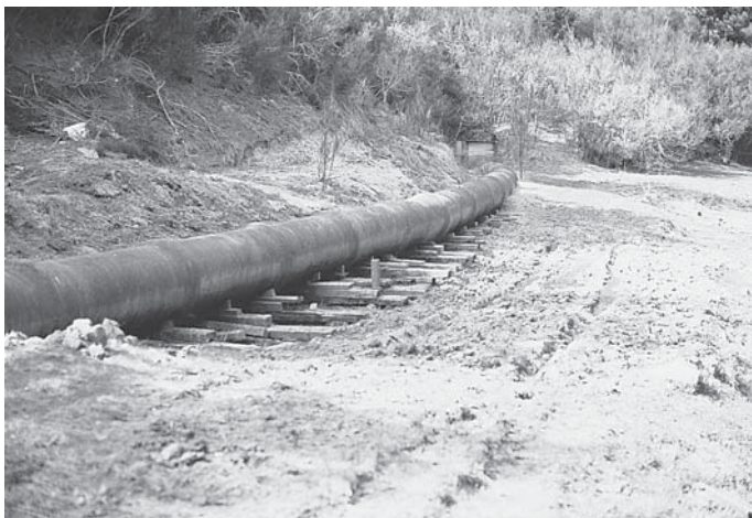
Silverstream Pipeline, showing jacking up - Civil Defence
