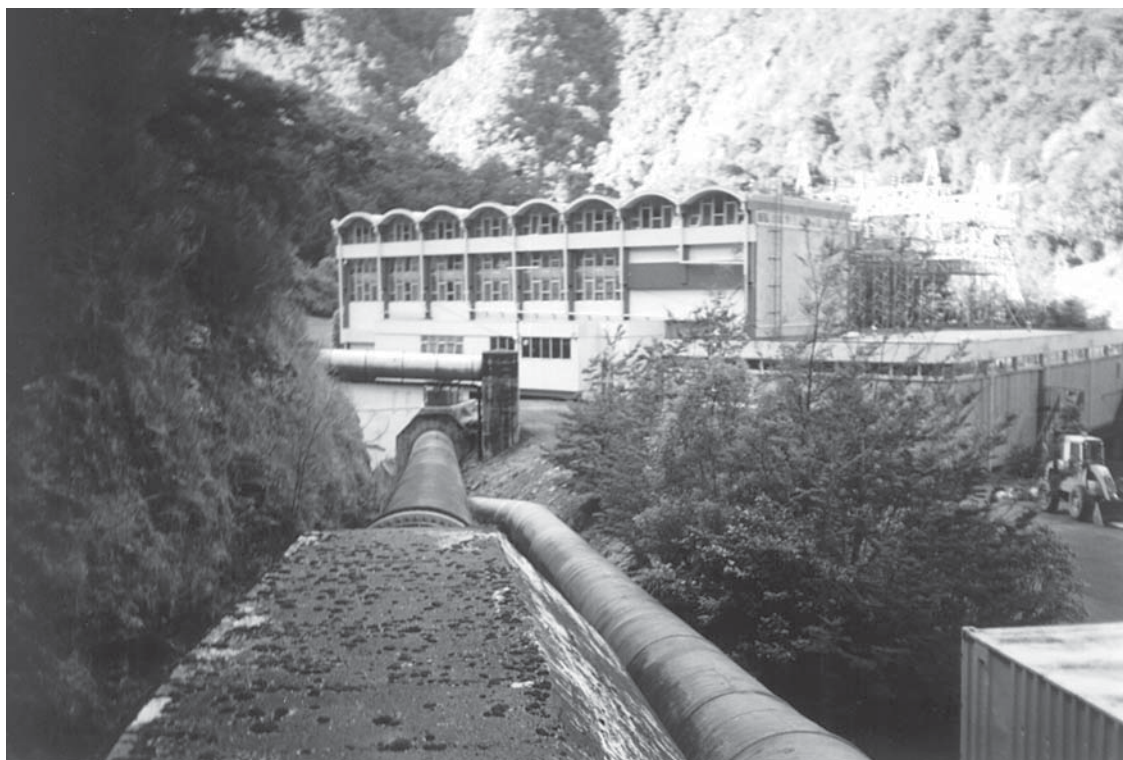
Penstock System Waipori 2A Station - Waipori Power Generator Ltd
