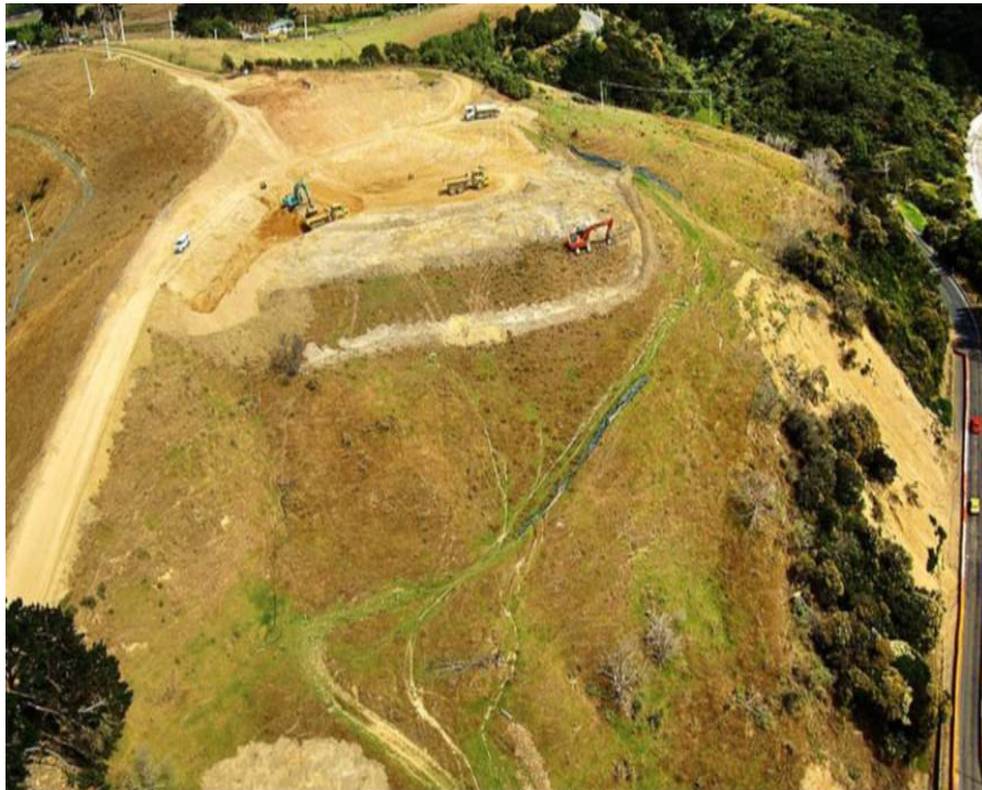
Figure 16. Remedial works to stabilise the landslide at Kawakawa Bay were well advanced in early February 2009. The measures used have included horizontal drains drilled into the lower slope, and extensive earthworks at the top of the landslide to unload the head of the slide, part of which required removal of a house built just below the headscarp. Source: Hancox, G.T., Nelis, S. (2009)
