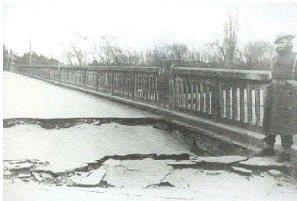
**Figure 2.8.** The approach to Masterton's Colombo Road bridge over the Waipoua River subsided 1/2 metre, so that traffic had to be diverted. Source: Alexander Turnbull Library.
