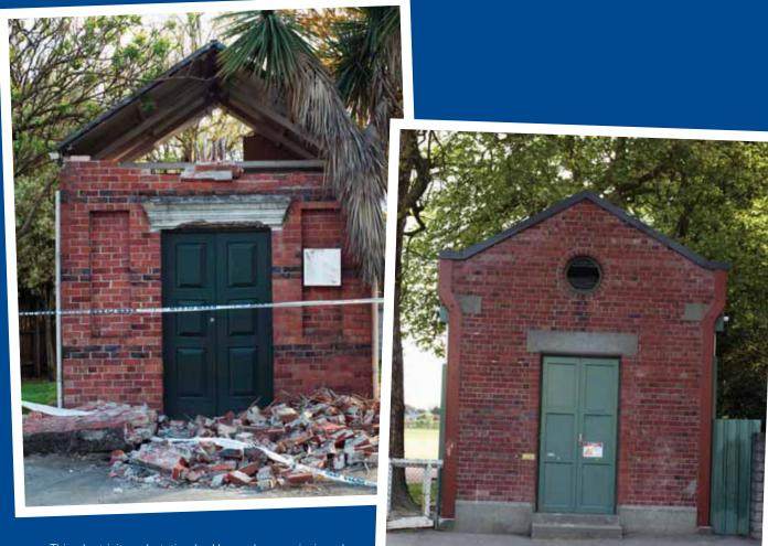
This electricity substation had been decommissioned prior to the earthquakes and was unstrengthened
