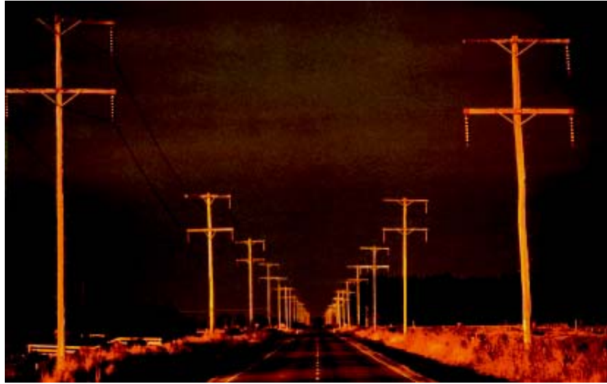
Single circuit poles carrying two single 110 kV circuits. While Transpower has over 17,000 such pole structures in service, the number is gradually declining as multiple single circuit transmission lines such as these are replaced with newer double circuit lines.
