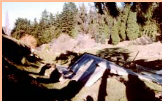
Compression ridges formed at the toe of the Sun Club Slide area. This deformation destroyed the swimming pool and tennis court (left), and also the badminton court (right). (Photos: Graham Hancox, GNS)
