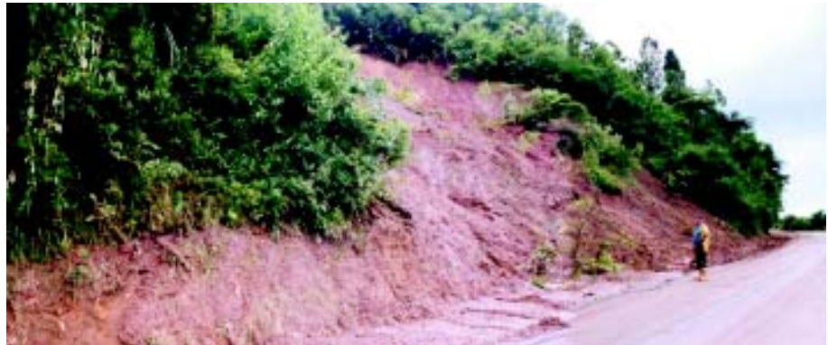
Fig 2: Main slip site (December 2001) following the removal of approx 2000m 3 of debris. Note that the remaining vegetation is well established and well rooted, but fails to provide adequate support for this highly altered volcanic 'glue' of surface and subsurface material in heavy rain events.
