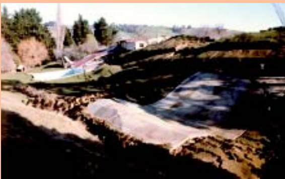
Compression ridges formed at the toe of the Sun Club Slide area. This deformation destroyed the swimming pool and tennis court (left), and also the badminton court (right). (Photos: Graham Hancox, GNS)
