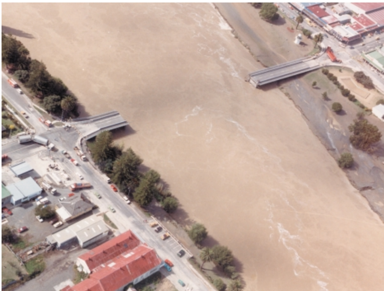
The missing Wairoa bridge, destroyed during the 1988 floods that accompanied Cyclone Bola (Photo – Daily Telegraph)
