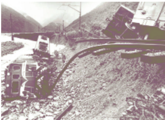
FIGURE 3: The Otira River, 22 May, 1980, after scour during a sustained flood destroyed the railway embankment. A locomotive driver was killed. (Photo: The Christchurch Press.)
