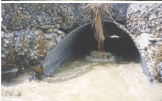
The Tinwald Burn outlet under SH6, north of Cromwell after the November 1999 flood event showing scour after overtopping of the road. (photo – Opus International Consultants Ltd)
