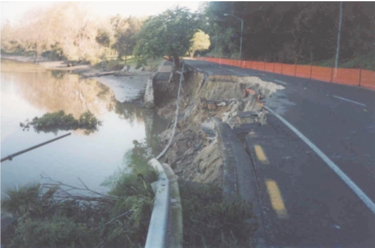
Failure of a section of Anzac Parade, SH 4 near Shakespeare's Bluff, Wanganui. This section dropped into the Whanganui River following the flood event in early October 2000. (photo – Opus International Consultants Ltd)
