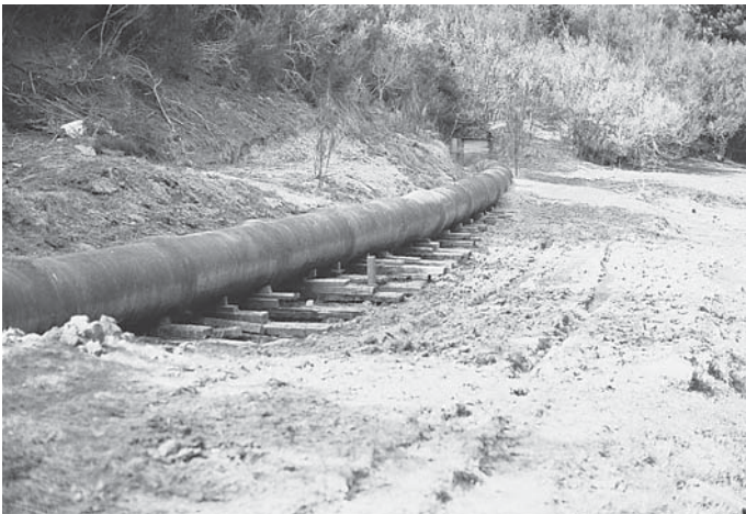
Silverstream Pipeline, showing jacking up - Civil Defence
