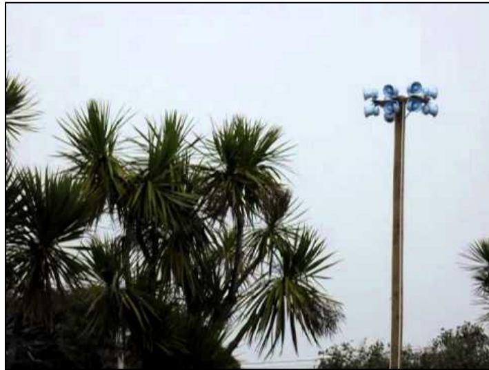
Figure 32: Array of horn-speakers to create an omni-directional array.
