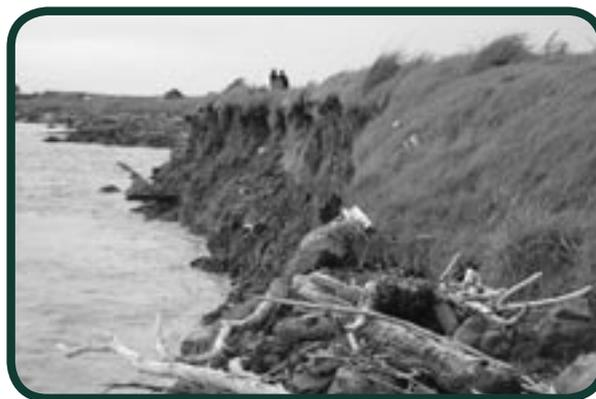
The changing river alignment resulted in erosion of the original stopbank.
