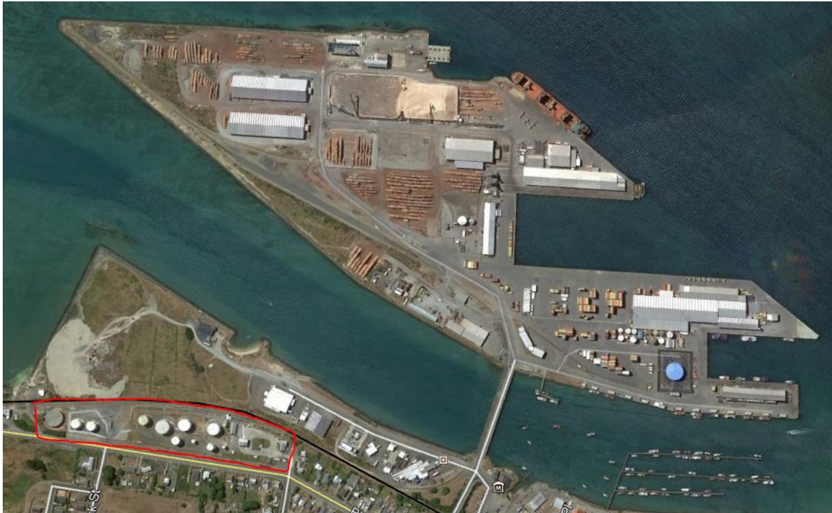
Figure 3 Oil Storage facilities SouthPort Bluff.
