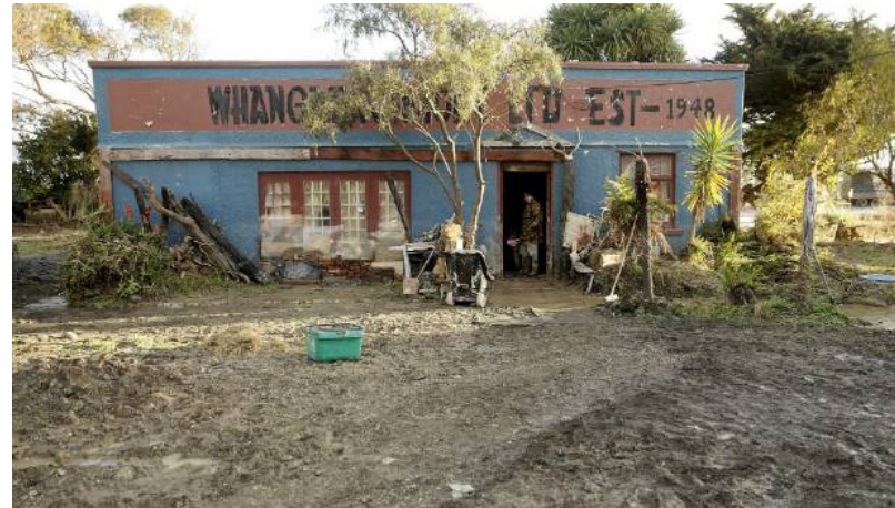
Figure 5: Post-flood clean-up in the Whangaehu Village after the 2015 flood (Source: http://www.stuff.co.nz/manawatu-standard/lifestyle/74829464/the-floods-that-came-with-force )
