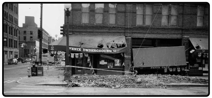
The brick parapet over the Fenix Cafe in Pioneer Square, Seattle, collapsed in rubble during the earthquake on 28 February.
