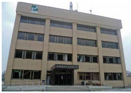
Example of a successful designated tsunami evacuation building in Kesennuma, Miyagi Prefecture, Japan. This office building was inundated to a height of 8 metres and sustained minor scour and non-structural damage. Videos show that people survived on the roof of this building.
