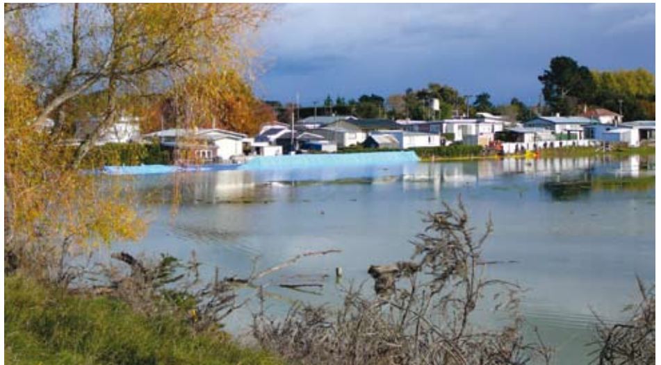
Waitaki Bridge settlement protected from flood waters by inflatable barriers
