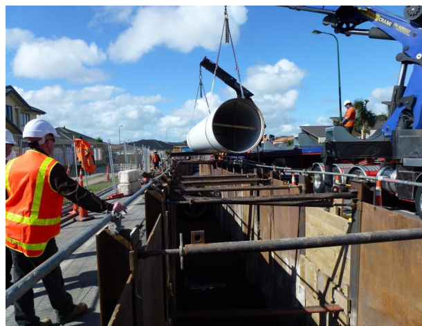
Installing 1900 dia pipe
