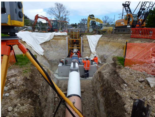
New Valve Chamber (Wiri 2 connection)
